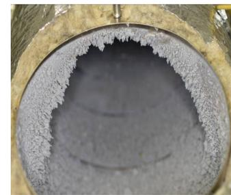
Fig. 7: Fouling of the flue gas duct – here the measuring section. Picture taken after only several hours of continuous operation.
