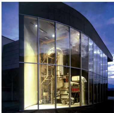
Picture 1: Power plant at municipal sewage plant
