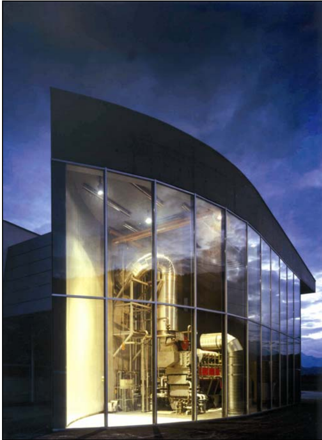
Picture 1: Power plant at municipal sewage plant
