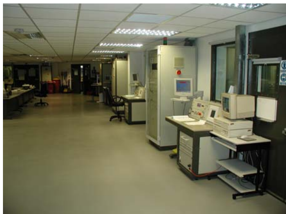
Figure 1 A bank of engine test cells at the Hazelwood laboratories
